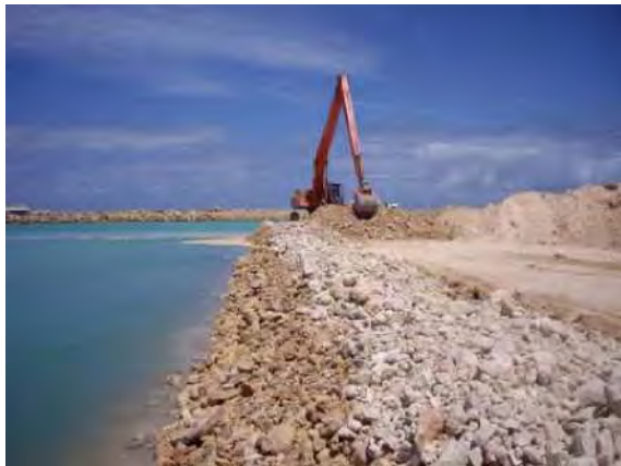
Figure 3: Placement of rock core bund
