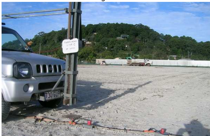
Figure 2: MASW site survey
