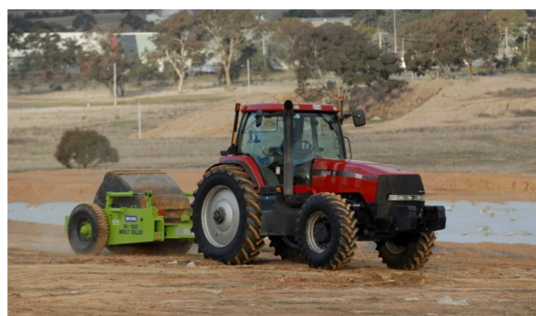
Fig.1 Four-sided impact roller towed behind a tractor
