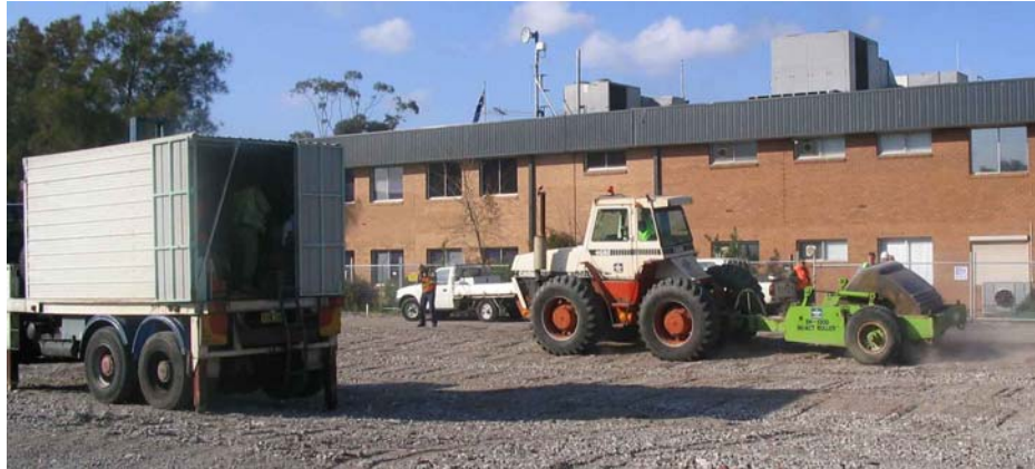
Figure 4. Facing south, impact rolling in progress. Note CPT rig on left, with geotechnical and vibration monitoring personnel near the southern boundary.
