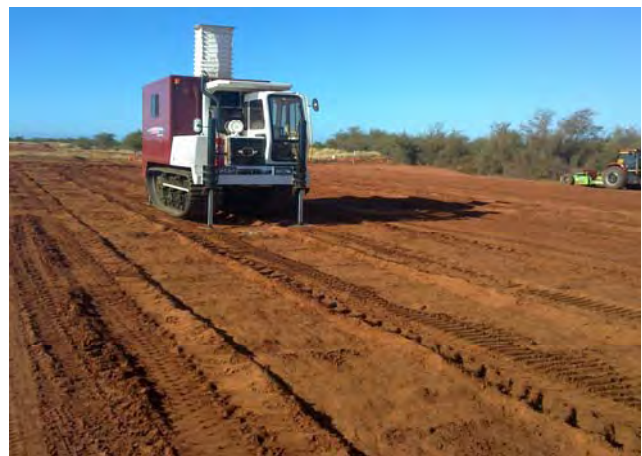
Figure 2. CPT rig undertaking post compaction testing
