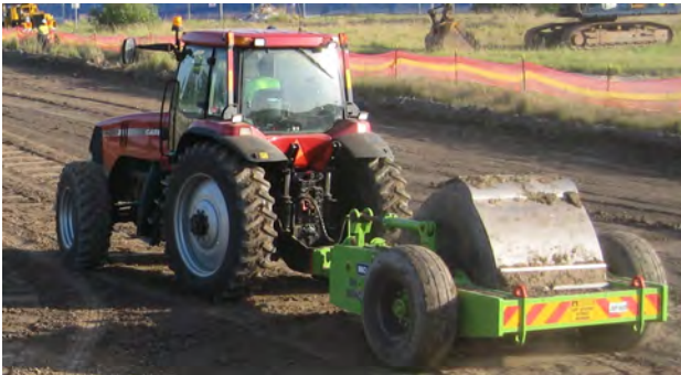
Figure 2. Impact rolling in progress.
