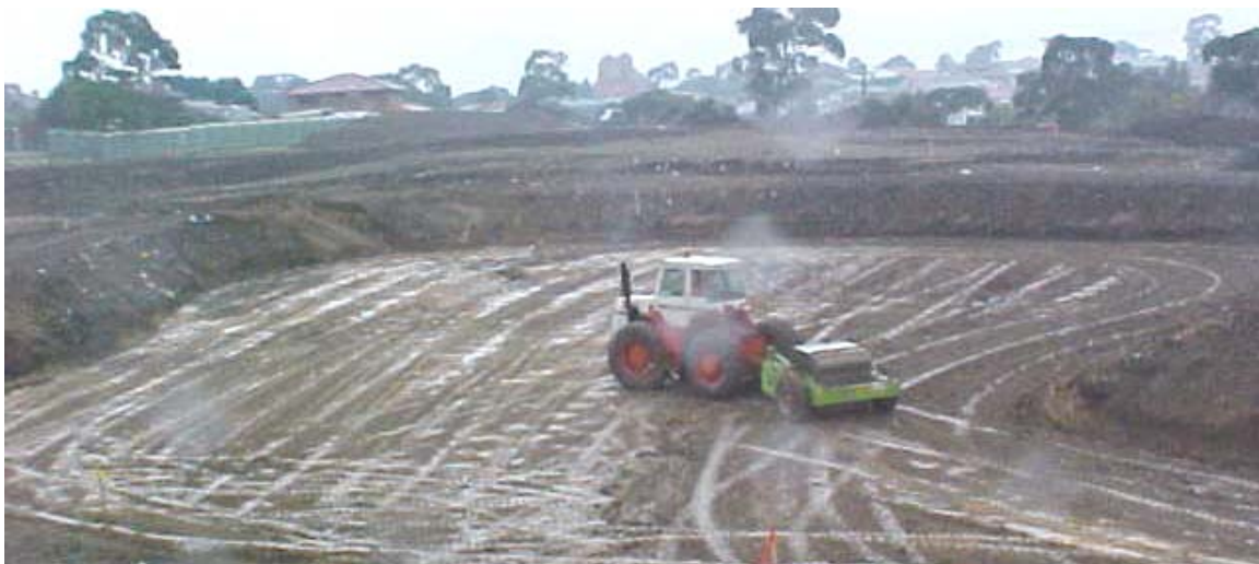
Figure 4. Impact rolling underway.
