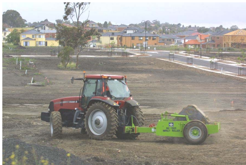
Figure 2. Impact Roller at a Melbourne residential development site.
