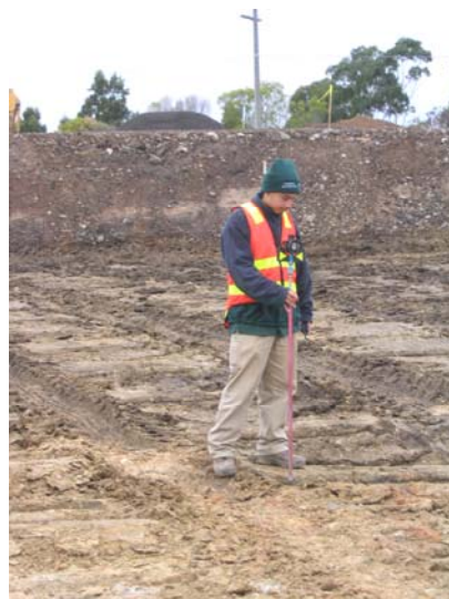
Figure 5. Monitoring of surface settlement during impact rolling.
