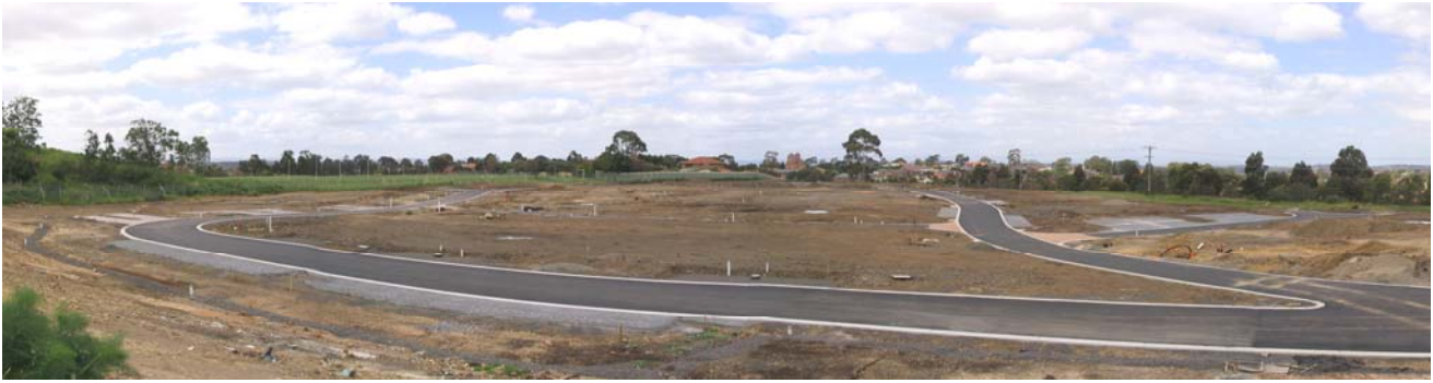
Figure 11. Earthworks, roads and drains nearing completion.
