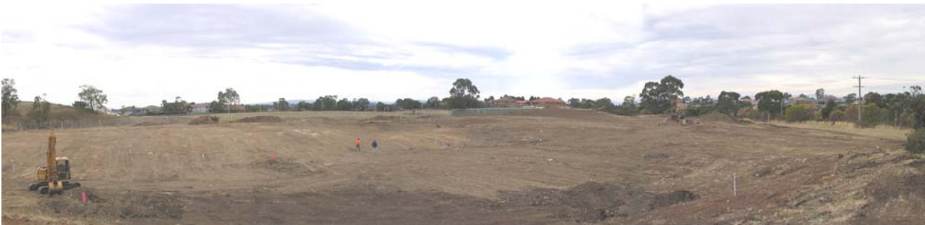
Figure 1. Panorama of depressed central area during preliminary site stripping.
