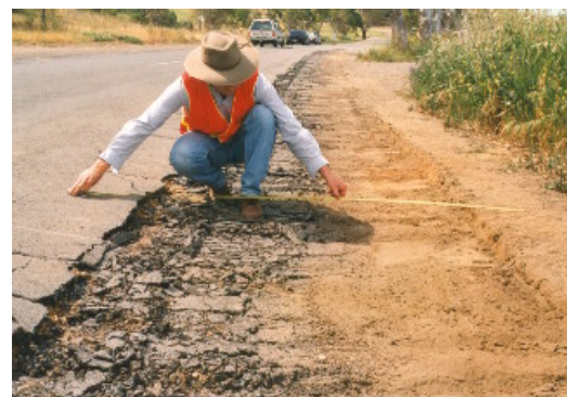
Figure 6: Settlement induced by impact roller.
