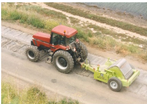
Figure 5: Road reconstruction in South Australia.
