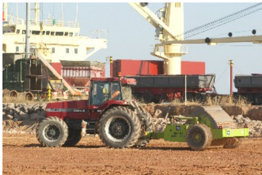
Figure 1: The "square" impact roller.
