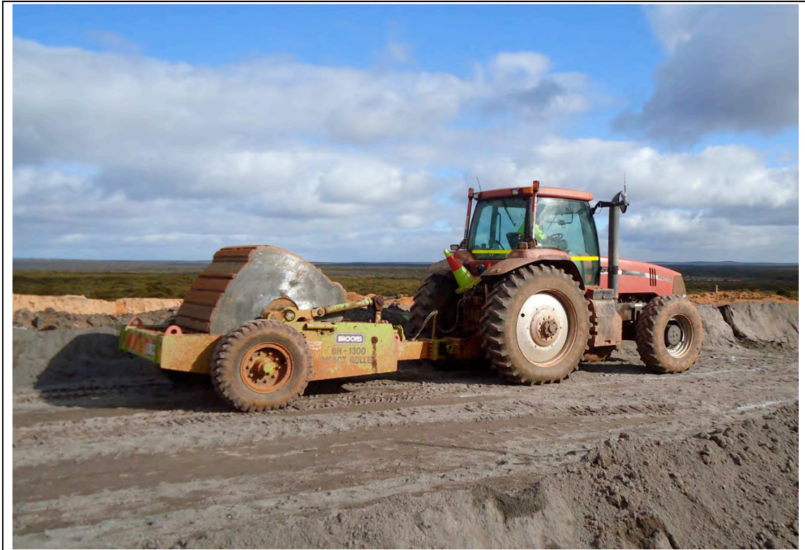
Photo 1 : Rolling dynamic compaction: Broons 4-sided 'impact roller'.
