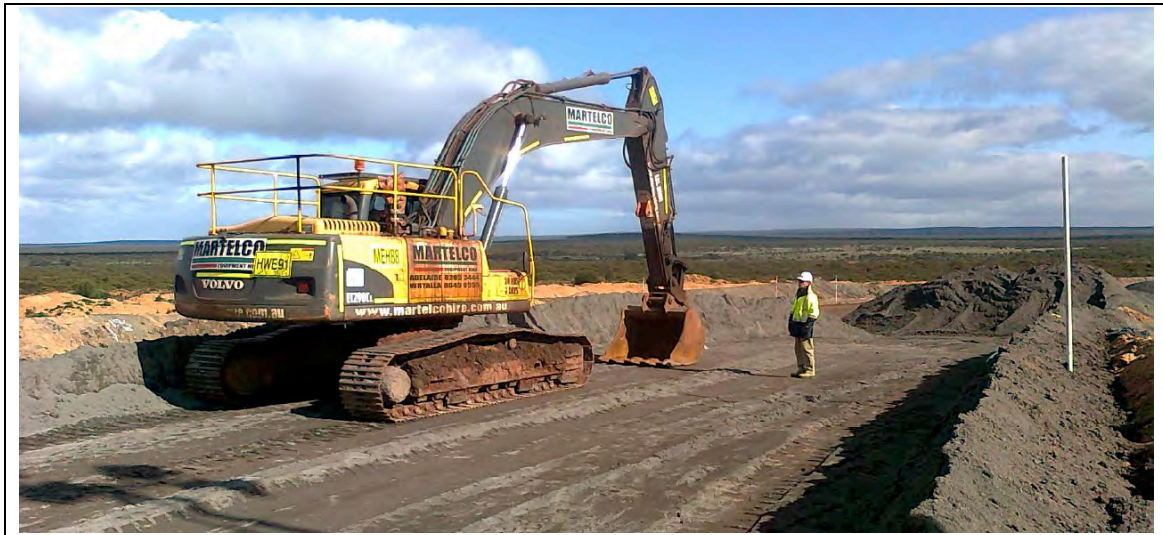
Photo 2 : Test pad construction showing excavator used.
