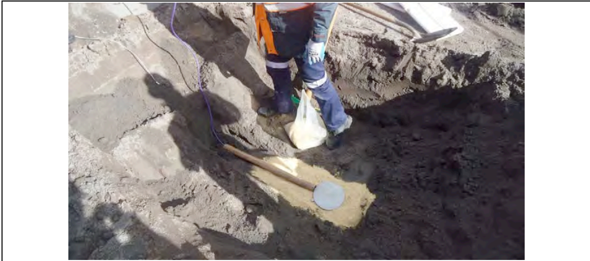
Photo 3 : Preparing the EPCs in situ on bedding sand.
