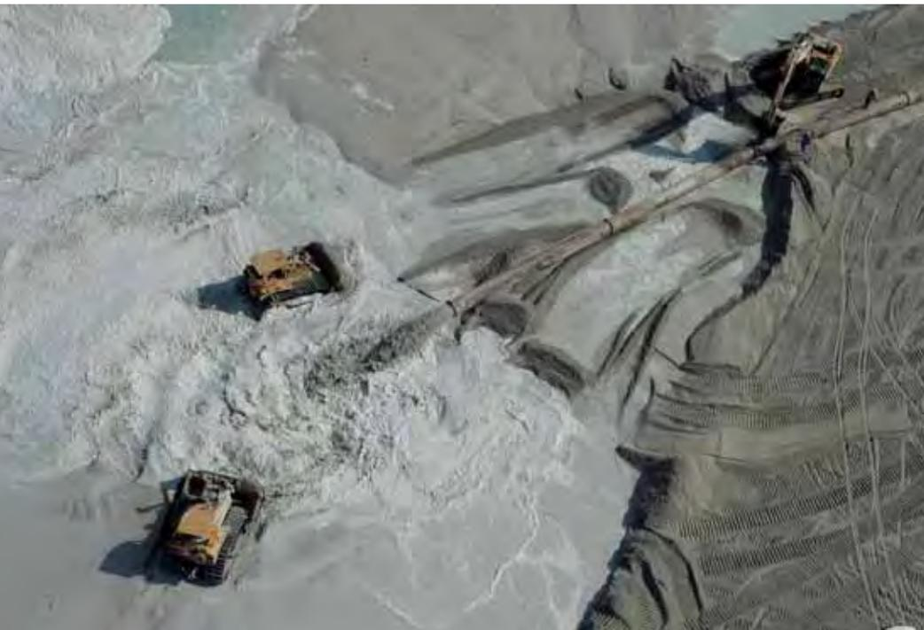
Figure 3. Initial compaction with bulldozers in front of the discharge pipe.
