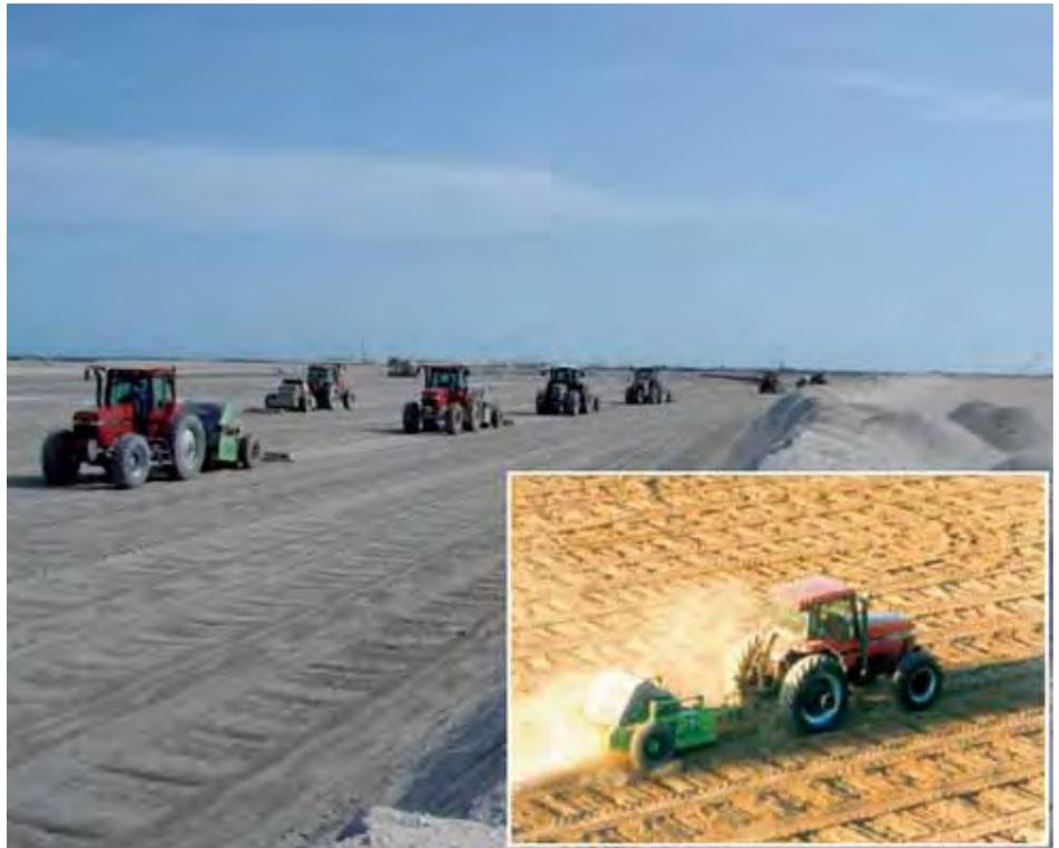
Figure 5. HEIC compactors on the NDIA project; right, a close-up of the compactor.
