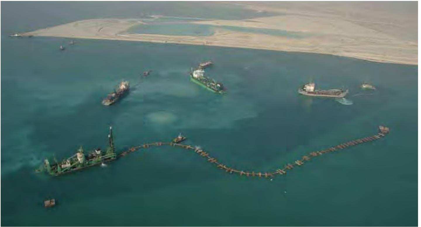
Figure 2. Dredgers at work in front of the reclamation area.
