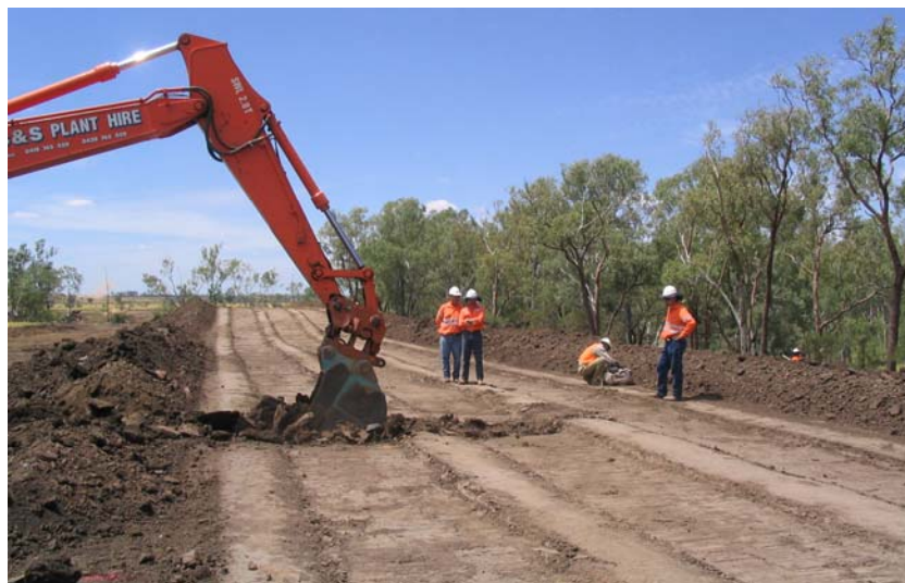
Figure 7: Trial embankment at Curragh North, Queensland.
