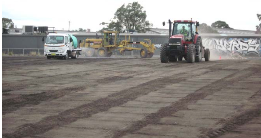
Figure 8: Trial underway on site in Sydney, NSW.
