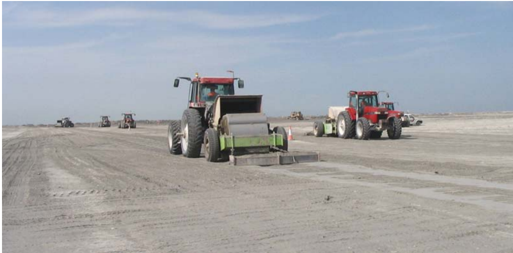
Figure 3: Impact rolling at the NDIA project, Qatar.
