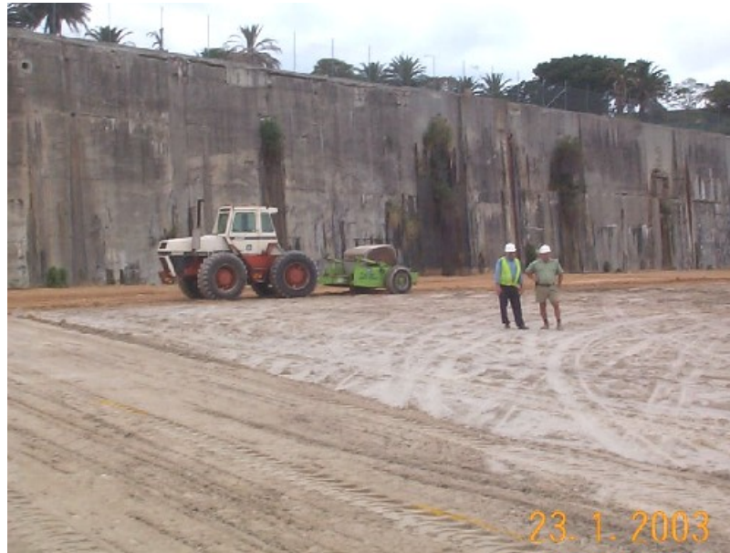
Figure 1: Impact Rolling in progress at the Bunnerong Site.
