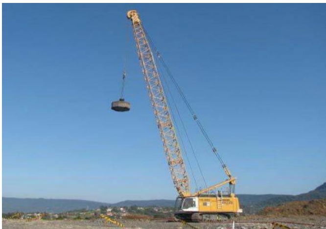
Figure 1. Deep Dynamic Compaction equipment.
