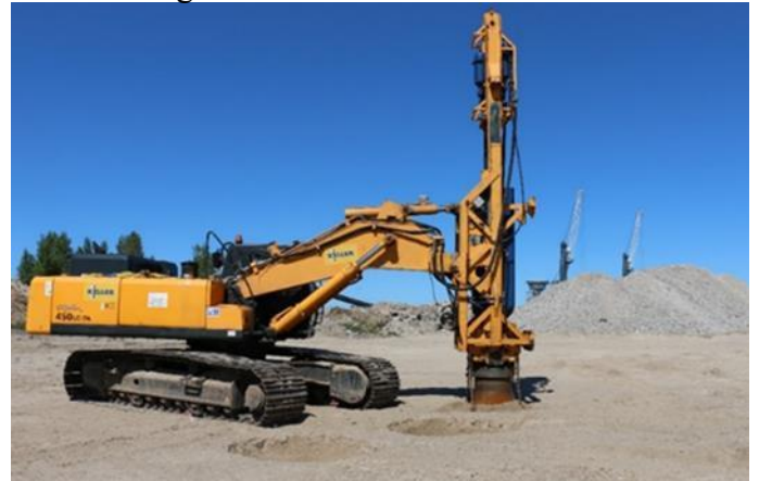
Figure 2. Rapid Impact Compactor.
