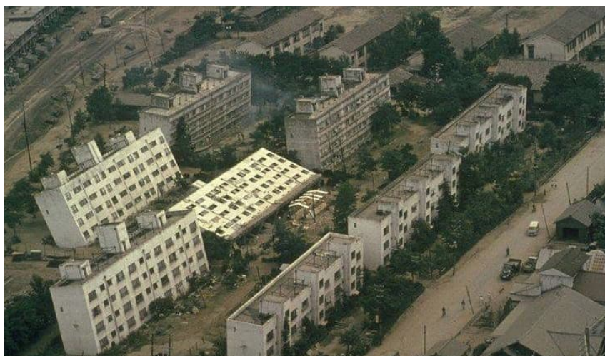
Figure 29: Foundation failure due to liquefaction as the result of the 1964 Niigata earthquake. (After Uni. of Washington 2000.)
