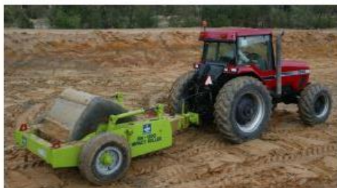
Figure 1. The 4-sided 'impact roller' towed behind a tractor
