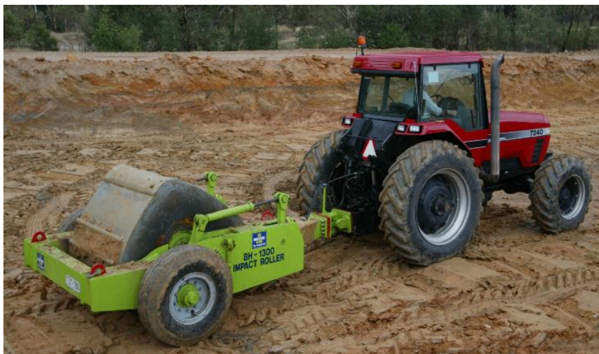
Figure 5.1 The 4-sided ‘impact roller’ and tractor.
