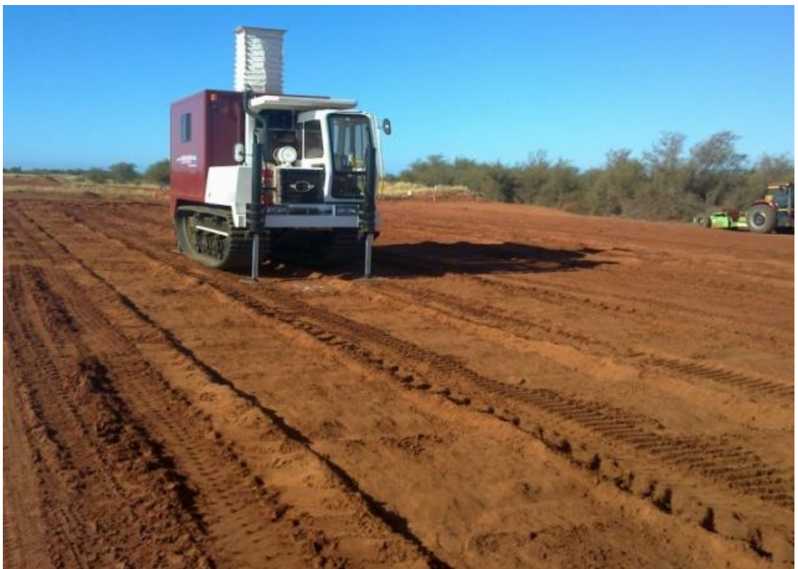
Figure 2. CPT rig undertaking post compaction testing
